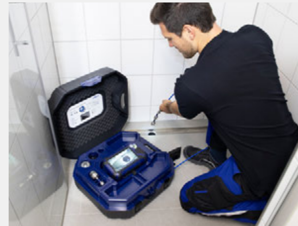
The waterproof camera head enables the inspection of sewers, among other things.
